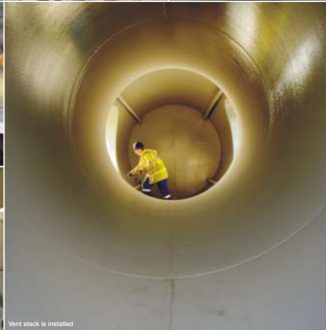
Vent stack is installed
