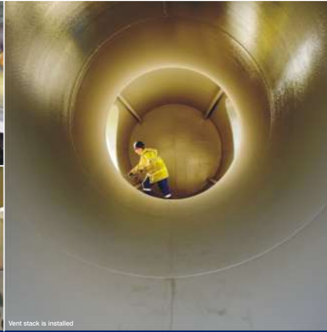
Vent stack is installed
