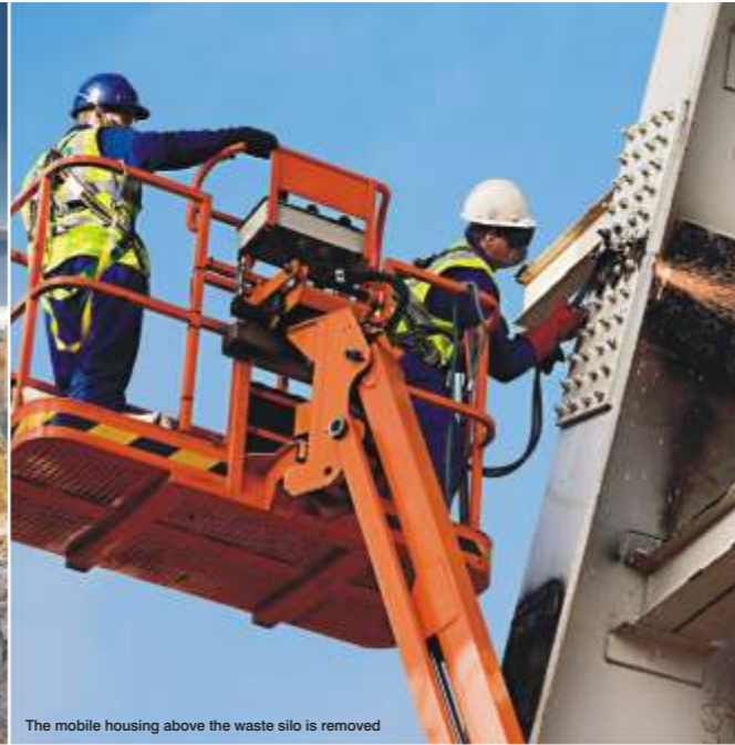
The mobile housing above the waste silo is removed
