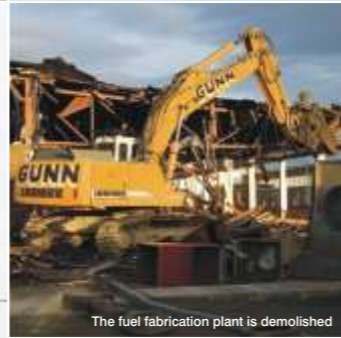
The fuel fabrication plant is demolished
