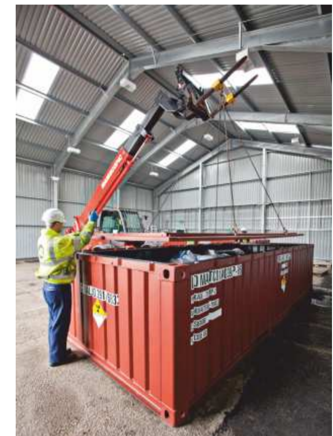
Much of the waste is low in radioactivity and can be buried safely in a series of engineered vaults being developed at the site.
