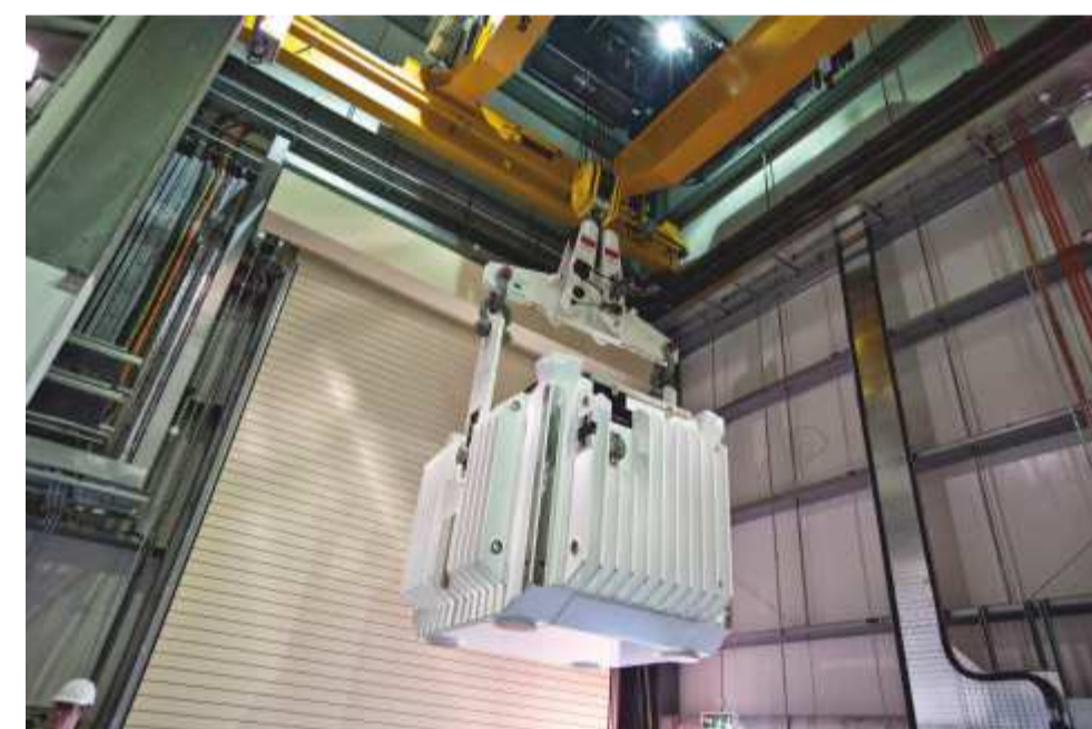
Robust containers known as flasks shield the more hazardous waste and fuels when it is transported
