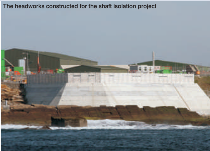
The headworks constructed for the shaft isolation project
