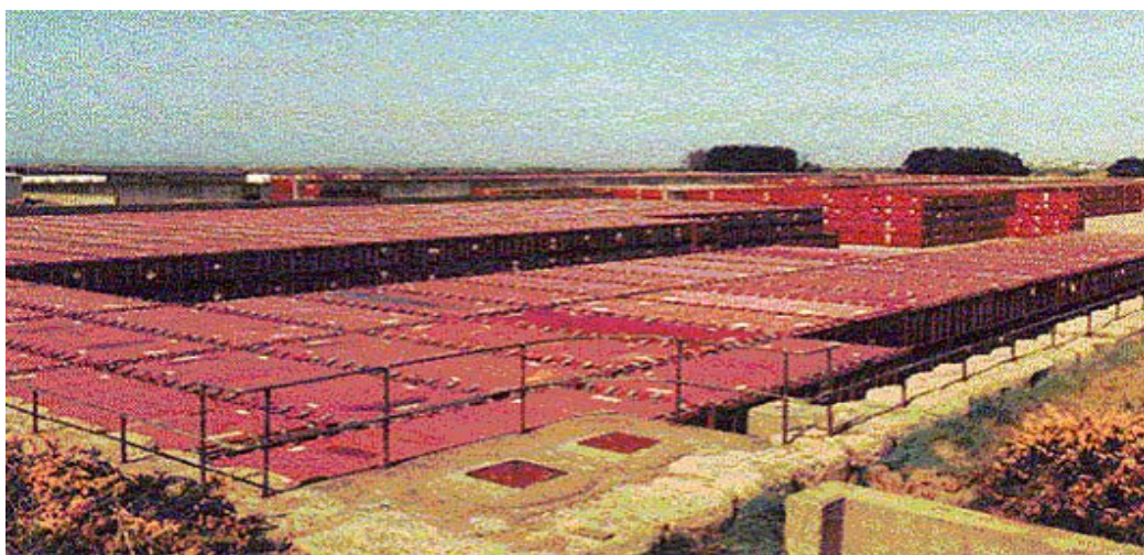
Photograph showing HHISO containers disposed of at the National LLW disposal facility near Drigg in Cumbria. Note that this differs from the proposed facilities at Dounreay in that this facility is being operated without a roof and is partly above ground.
