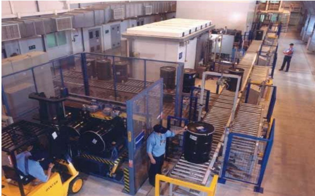
Photograph of the interior of the Downreay Waste Receipt, Assay, Characterisation & Supercompaction facility, showing inspection of LLW drums.
