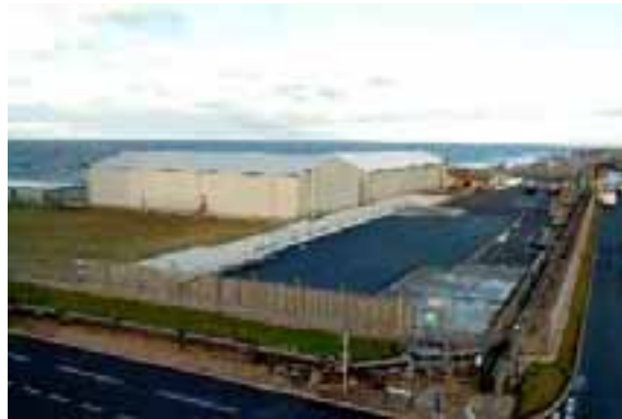
Figure 1. The existing Dounreay LLW disposal facility
