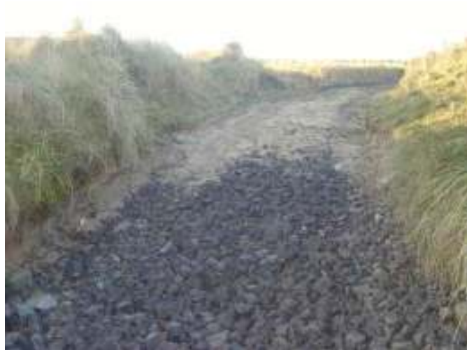
Figure B-2: Repaired Sandside path
