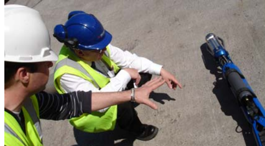
Bill Thompson, DSRL inspects pipe-crawler
