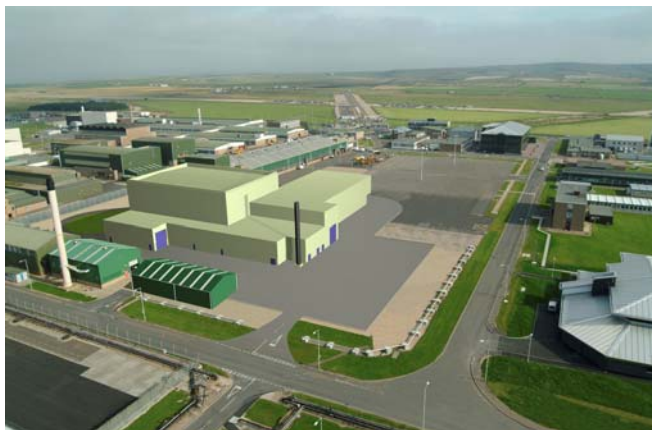
Figure 17: RHILW Immobilisation & Encapsulation Plant (RHILW-IEP)
