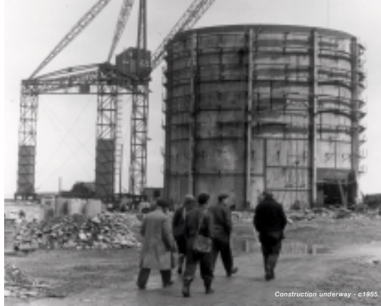
Fitting out of the Reactor Vault.
